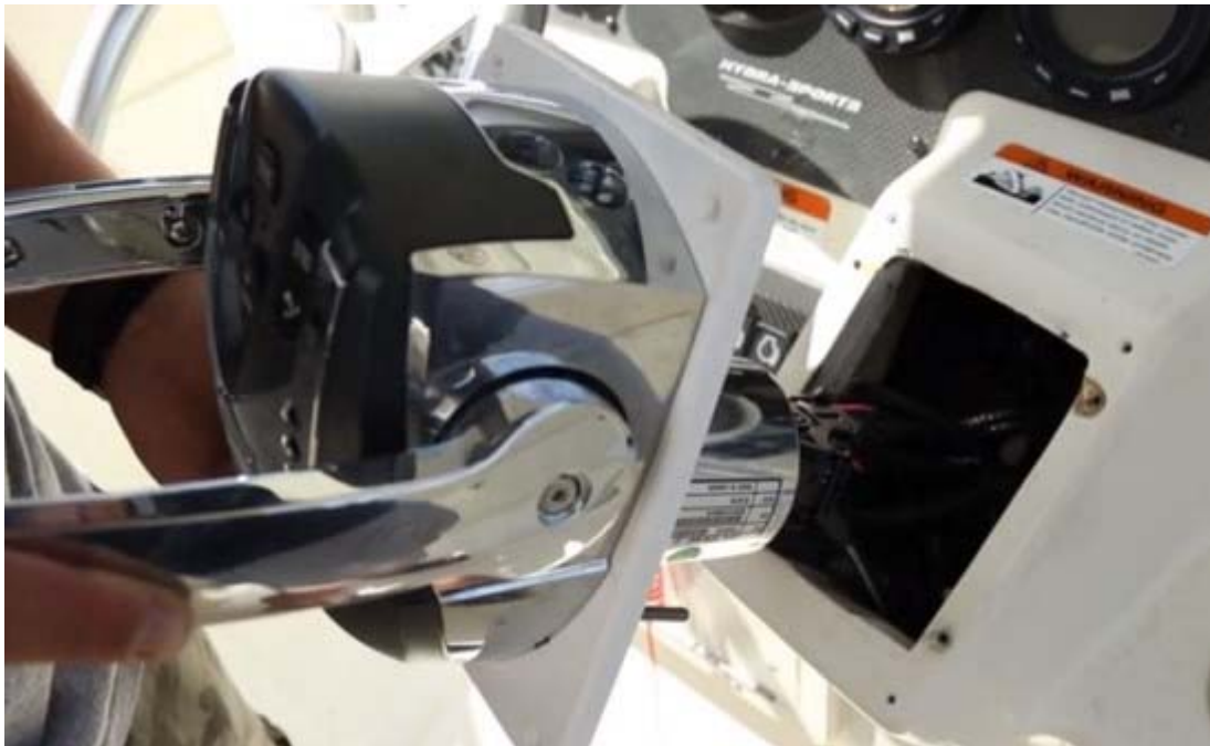
The new digital shift and throttle binnacle control is installed with wires running from it instead of cables.
